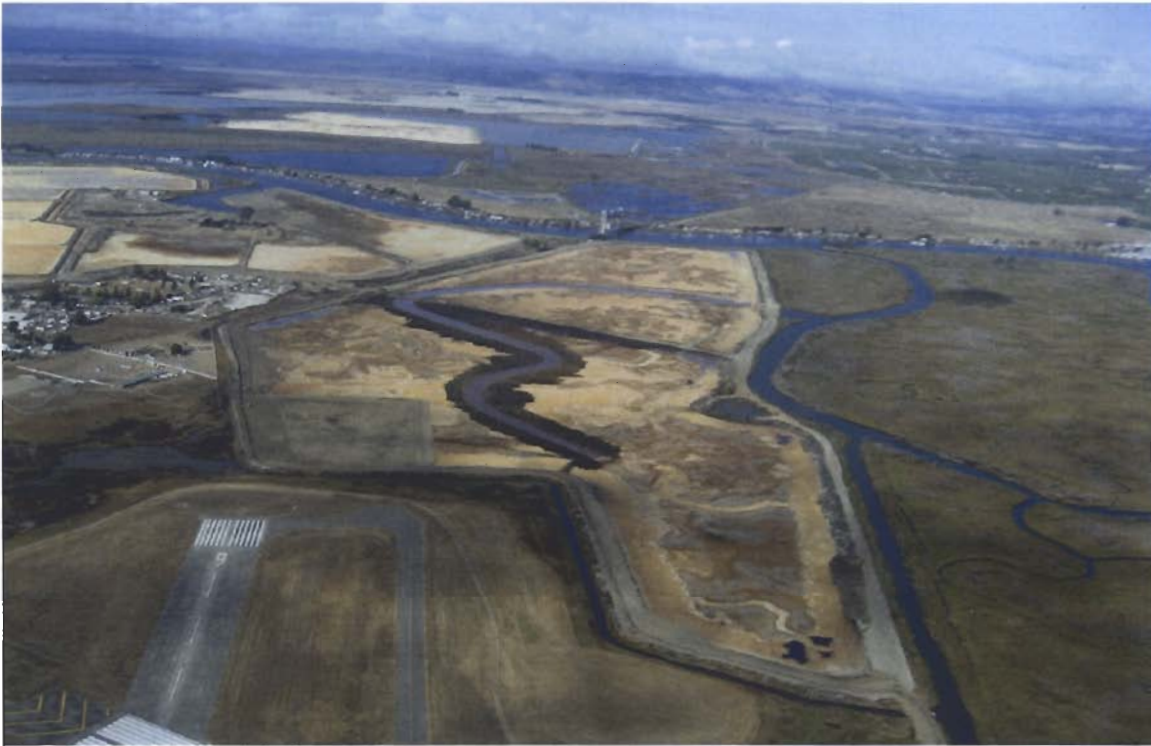
Figure 2. This aerial view clearly displays the reconstructed historic channel before the NUB was breached. Photo Courtesy The Dutra Group, September 2008.
